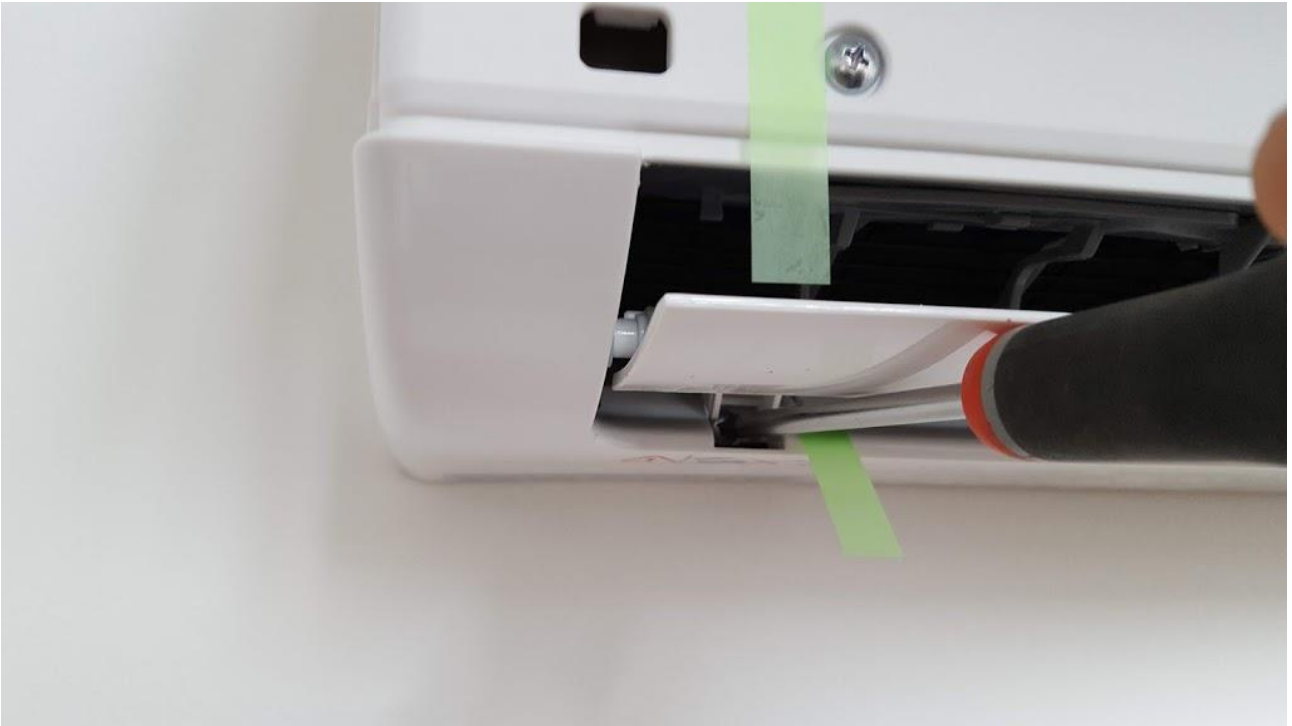
Lossa strömkoppling till front panel
